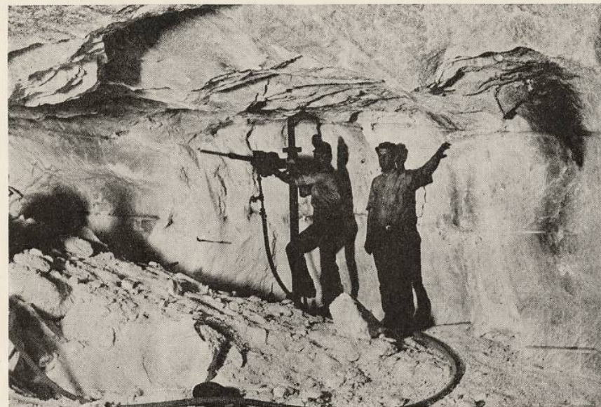
FIG. 6—700 feet down! Drilling holes preparatory to blasting out solid salt with dynamite at the Morton Salt Company's Kleer mine near Grand Saline, Texas.
