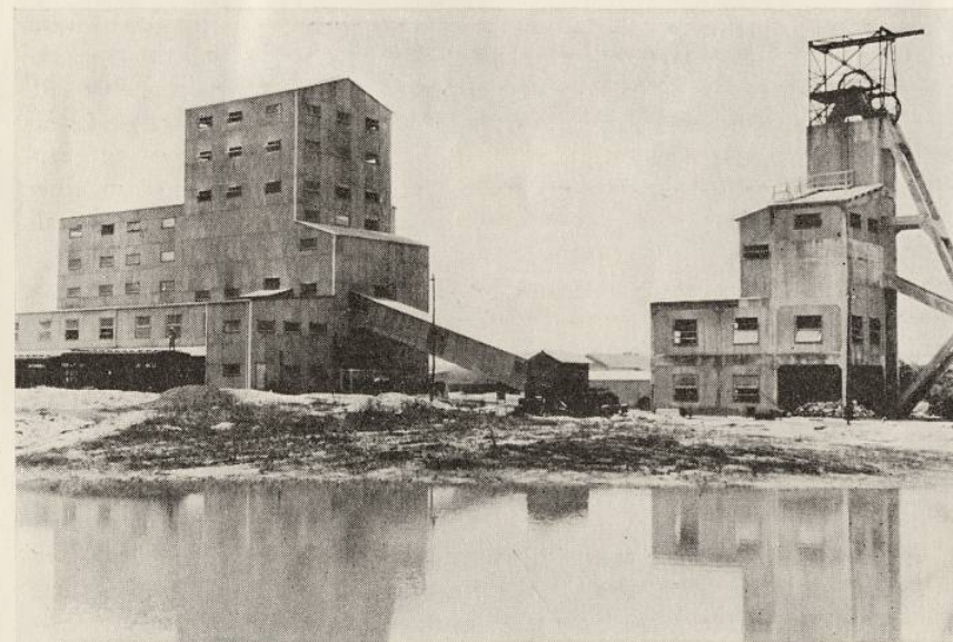
FIG. 7—Surface buildings of the Morton Salt Company's Kleer mine. That at the left is the "tipple," containing the crushers, screens, etc., while that at the right tops the elevator shaft of the mine.
