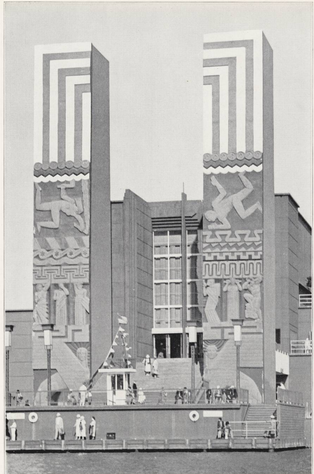
The Water Gate—Electrical Building
