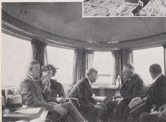
The solarium, at the rear of the train
