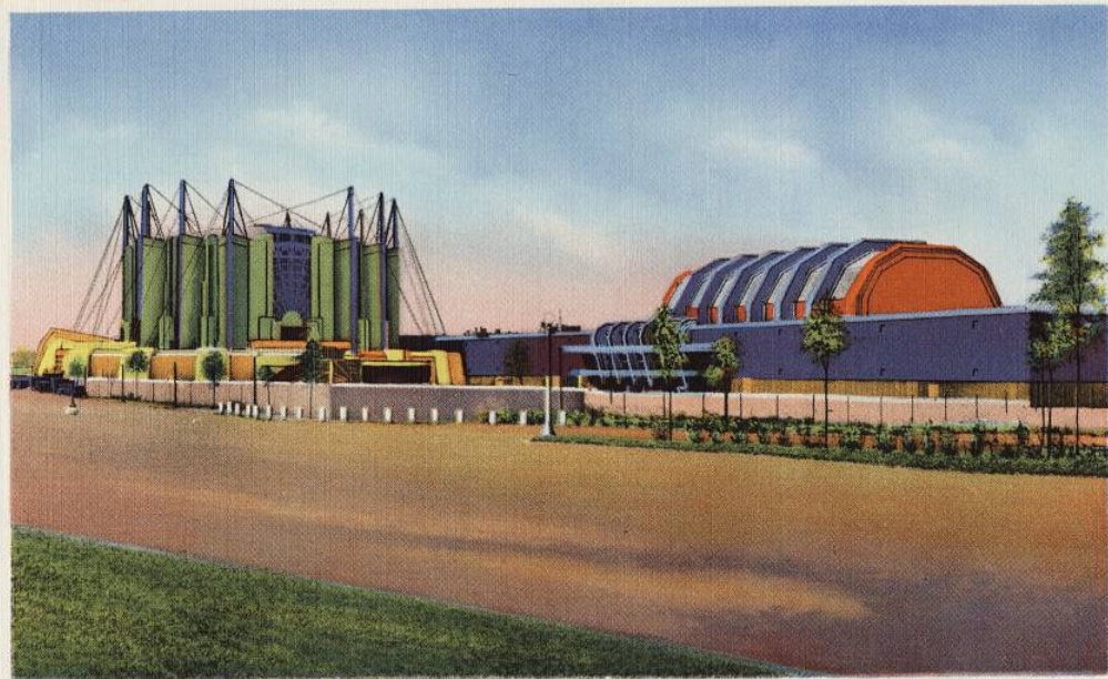
Travel and Transport Building
