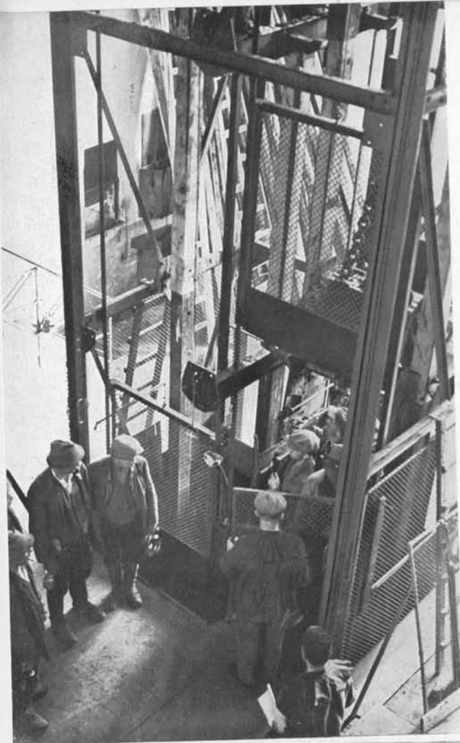
Hoisting equipment Concord Mine
