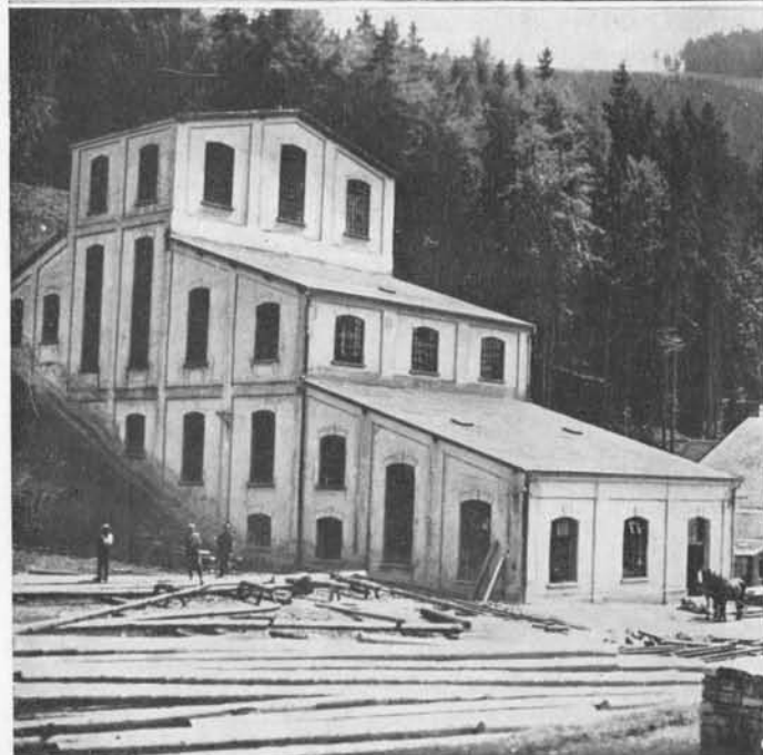
Mining pump ● Ore Dressing Department at the "Saxon Noblemen" Mine
