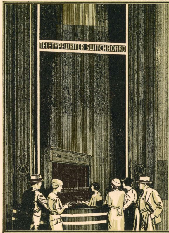
Exhibit 2B. Teletypewriter Switchboard
