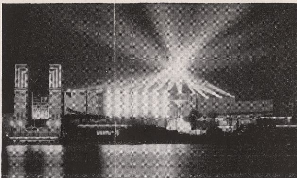
The Electrical Building at A Century of Progress
