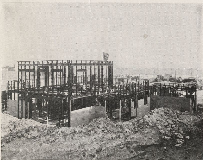
In this frame of steel is a new romance in building. The steel framework is put together with nails by carpenters.
