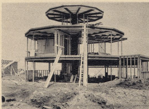
Steel and concrete work finished
