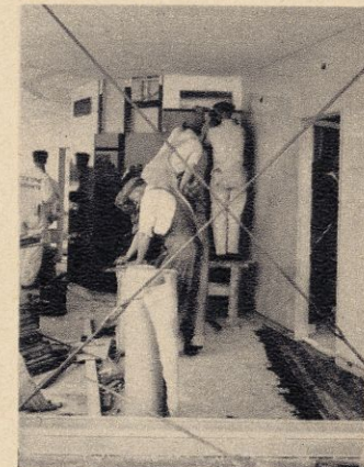
Setting interior glass walls
