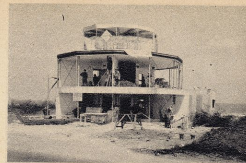
Glazing and installing partitions
