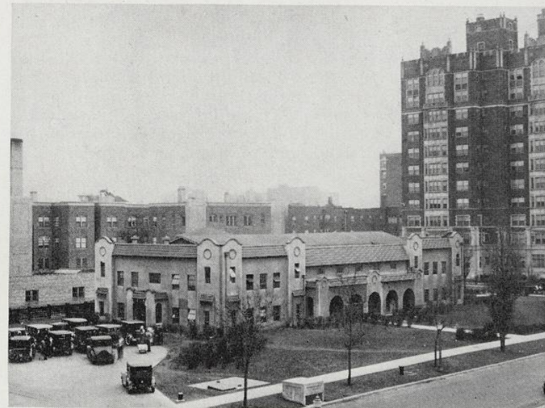
Figure 22—Experimental Filtration Plant
