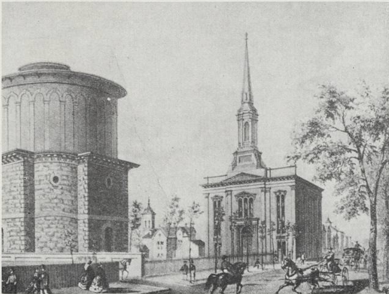
Figure 16—Old Reservoir at Monroe and Morgan Streets—1858
