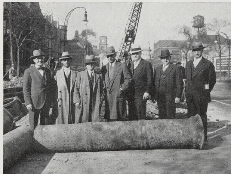
Figure 19—Section of 24-inch cast iron main laid in 1854 and removed in 1932
