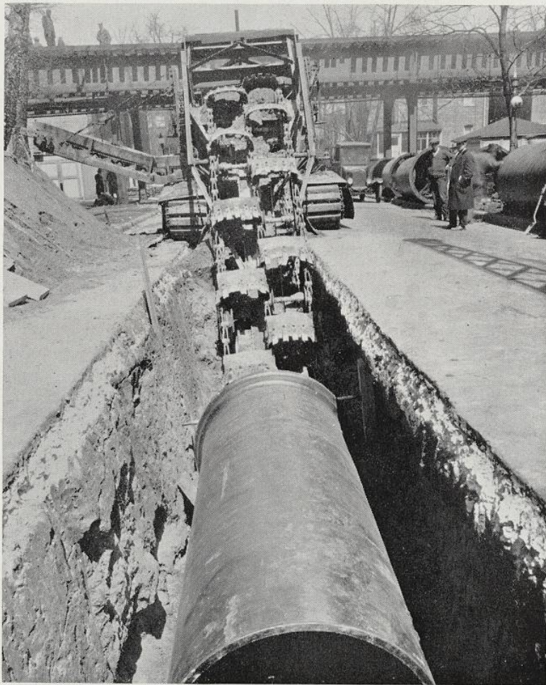
Figure 20—Laying large water main
