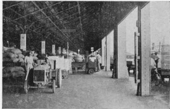
Cargo-handling on one of the steel and concrete piers at Cristobal.
