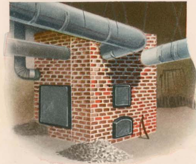
One of the first warm air furnace installations
