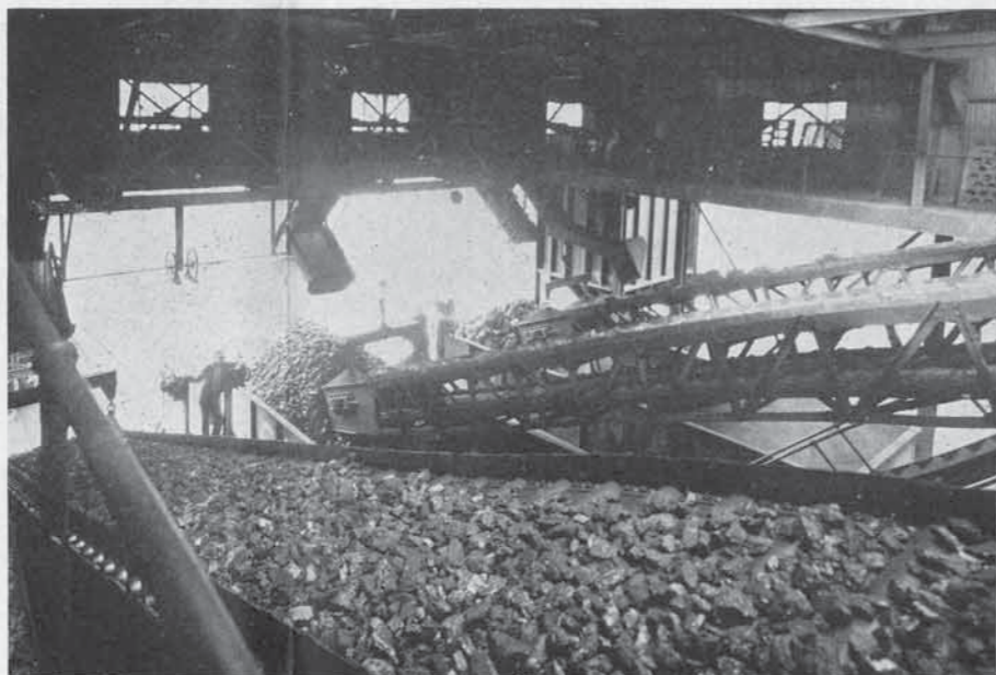
FROM THE TIPPLE THE COAL SAFELY CREEPS DOWN A CONVEYOR TO THE RAILWAY CARS BELOW
