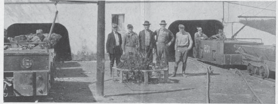
TYPICAL ENTRANCE TO A MODERN MINE Empty cars enter at the right and emerge loaded at the left
