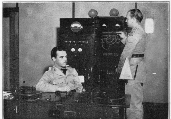
RADIO CONTROL ROOM—SCHOEFIELD BARRACKS, T. H.
