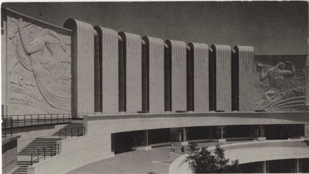
ABOVE ELECTRICAL COURT. THE TWO BAS RELIEFS ARE INSCRIBED TO "LIGHT, THE BEGINNING OF ALL THINGS" AND "ENERGY, SUBSTANCE OF ALL THINGS." A CENTURY OF PROGRESS INTERNATIONAL EXPOSITION, CHICAGO.
